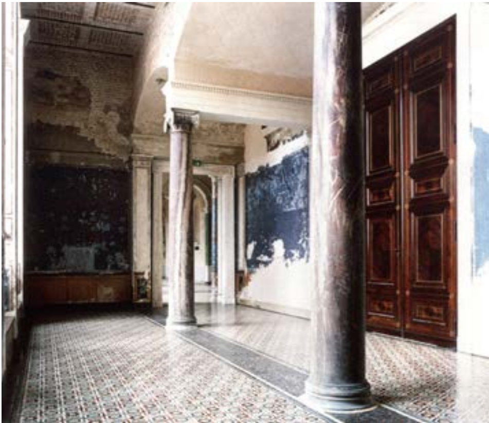
Top: Neues Museum, the restored floor contrasts with the unrestored decor (Neues Museum Berlin, 2009)
